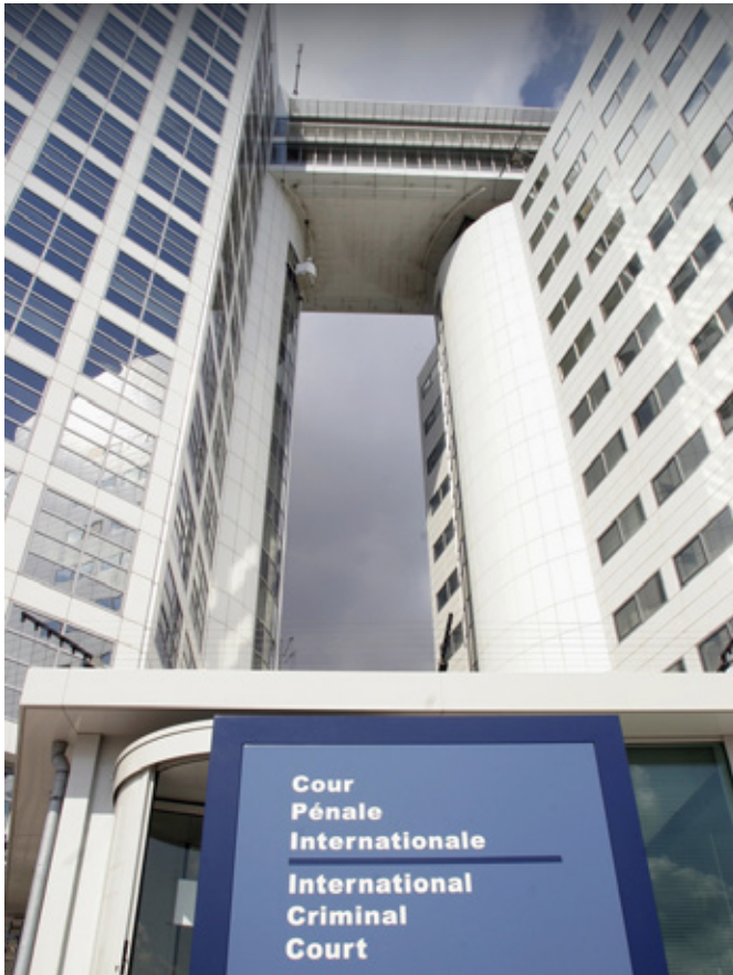
The main entrance of the ICC's Headquarters in The Hague, The Netherlands ©ICC-CPI / Wim Cappelen
